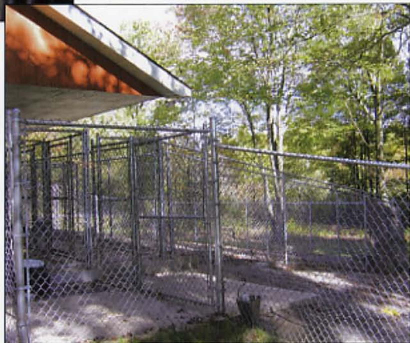
This page: MYNE Kennels utilizes indoor-outdoor runs with guillotine doors.
